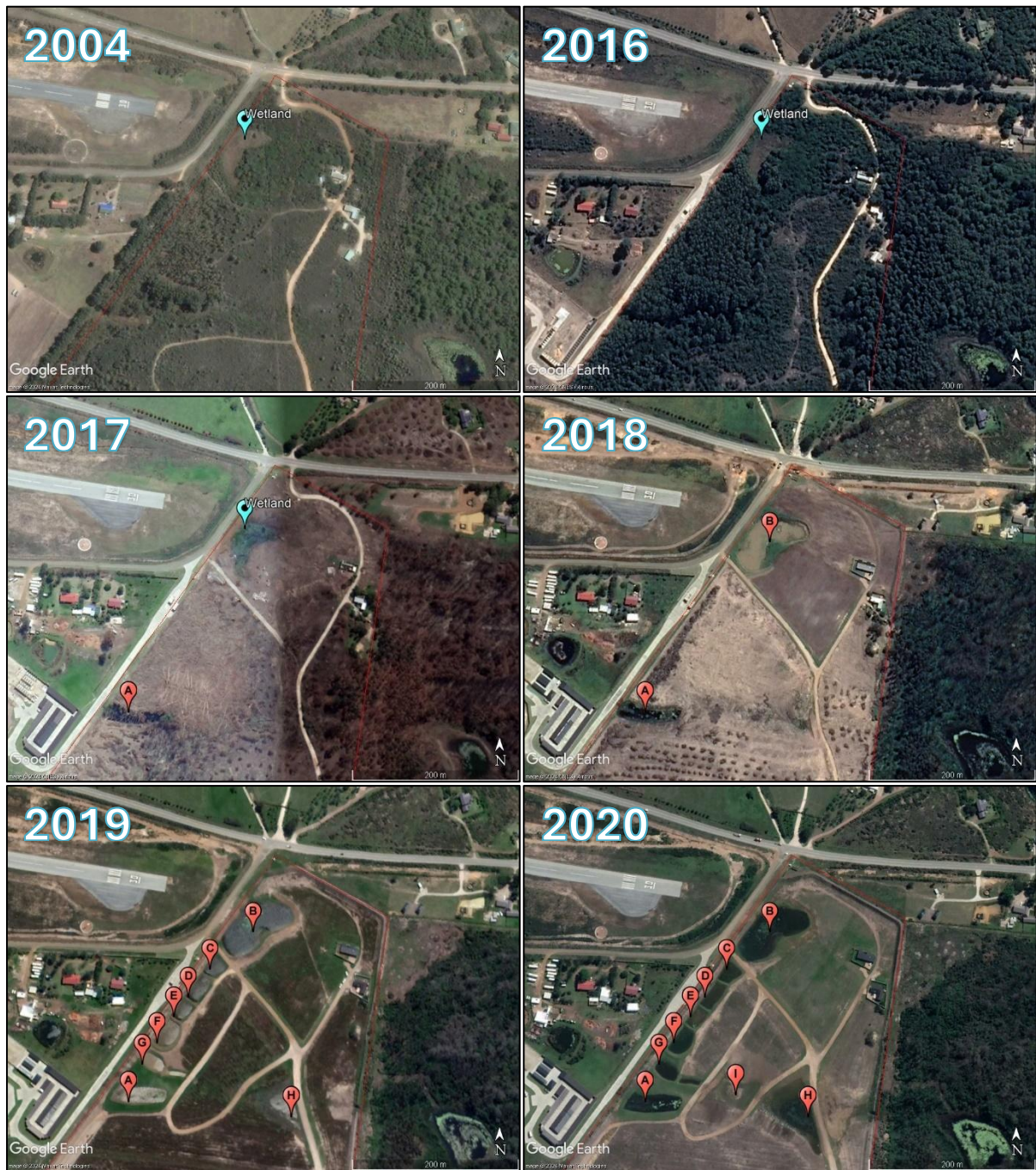
Figure 6: Google Earth imagery indicating the progression of the construction of dams on the property.
