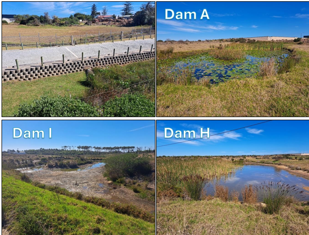
Figure 8: View to the west of Dam A, showing the road adjacent to the property. A stormwater channel is visible to the west of the road as well as a 600 mm pipe which discharges water from the channel into Dam A (top left); Dam A; Dam I; and Dam H.
