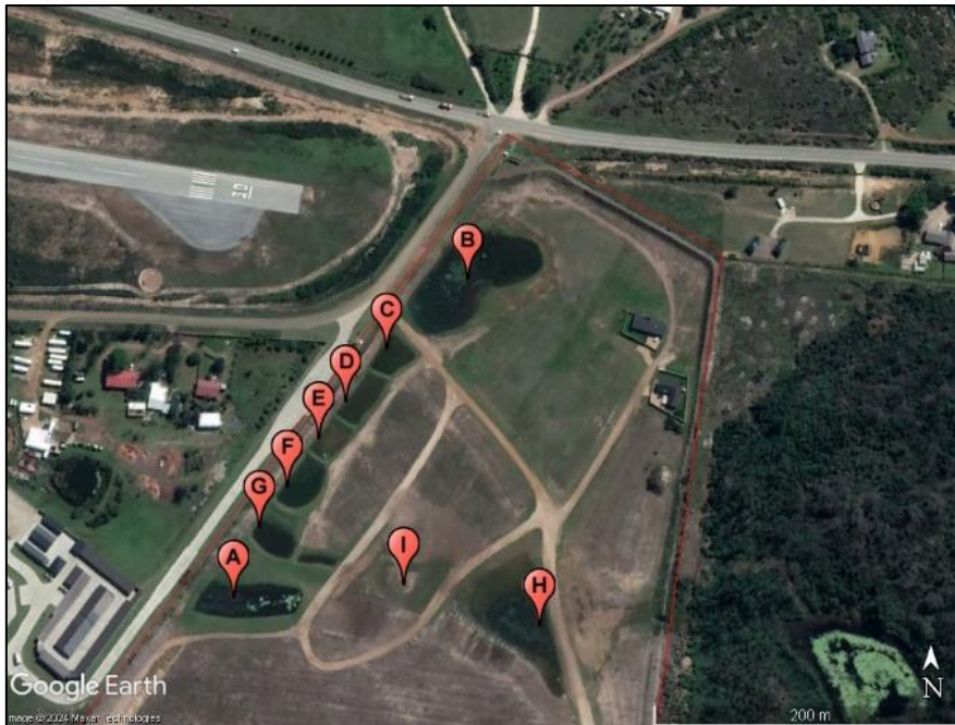
Figure 4: Dams present on Erf 8010 prior to their removal.
